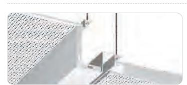
Partition receiving profile with built-in drop to accomodade height difference between a corridor and an office area.
