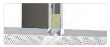
Metal ceiling with beam grid installation and sound barrier. For lateral attenuation between rooms.
